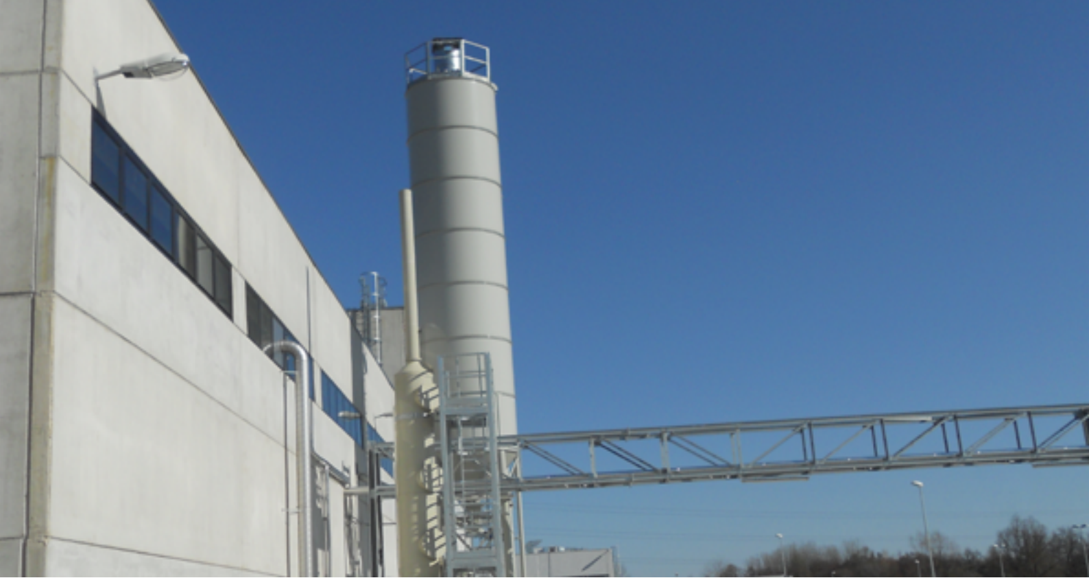
sopra, Pipe-rack Impianto tecnologico up, Pipe-rack technological system
