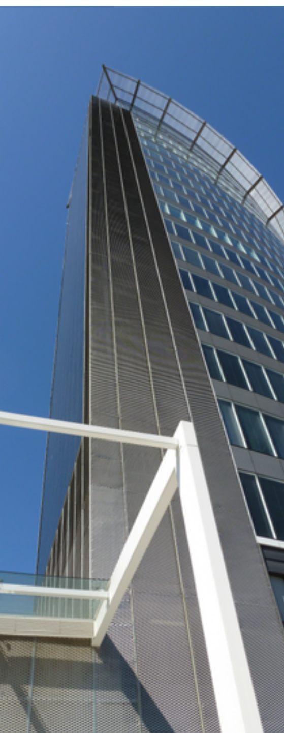
Vista torre Tower view
