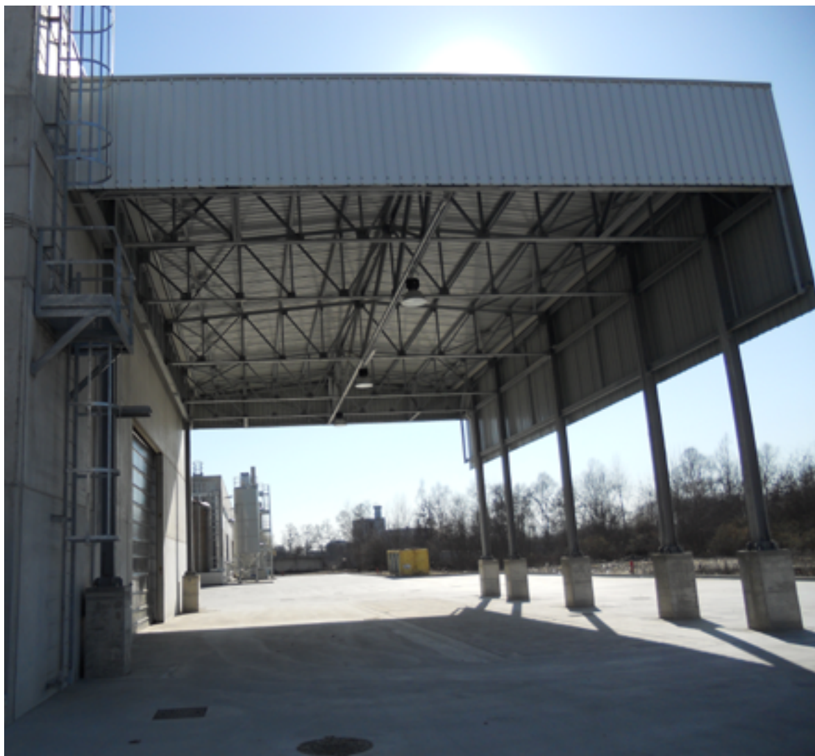
sotto, Pensilina carico-scarico down, Canopy loading and discharging system
