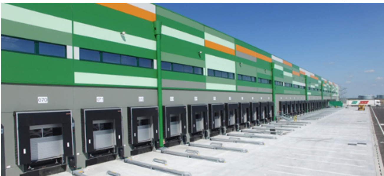
Stabilimento, vista esterna Building, external view
